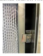
To replace the HEPA filter ensure that the gasket on the HEPA filter faces inwards toward the flange, slide the filter in place along the filter guides and re-install the filter tabs and filter tab securing nuts. Tighten the tabs so that the gasket is compressed approximately ½ of the thickness. This allows for the filter to be reseated and tightened at a later time if necessary.
